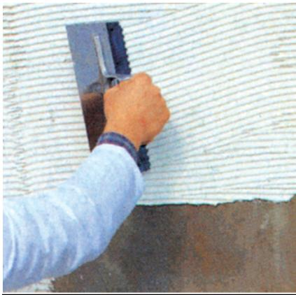
1. Cover and flatten the wall with a thin set approved for use with a glass mosaic tile. We recommend latex modified thin set (mix the powdered thin-set mortar with latex additive in bucket) that can easily be found in most home improvement stores such as Home Depot or Lowes.
