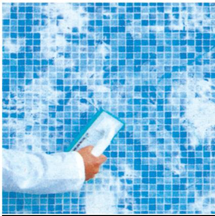
4. After taking off the paper of the mosaic sheet, level up the joints with white grout.
