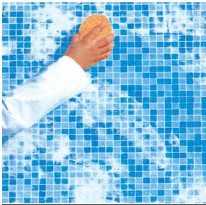
5. Clean up the remaining grout and adhesive on surface with a soft cloth and tissue.
