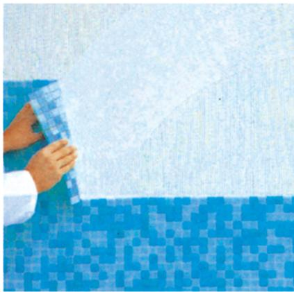
2. Before laying the mosaics, a thin layer of cement mortar should be pasted to the cover surface. Then, fill the joints between each small mosaic on the net with white mortar paste, press the mosaic sheet toward the wall in accordance with the direction of the arrow on the setting paper.
